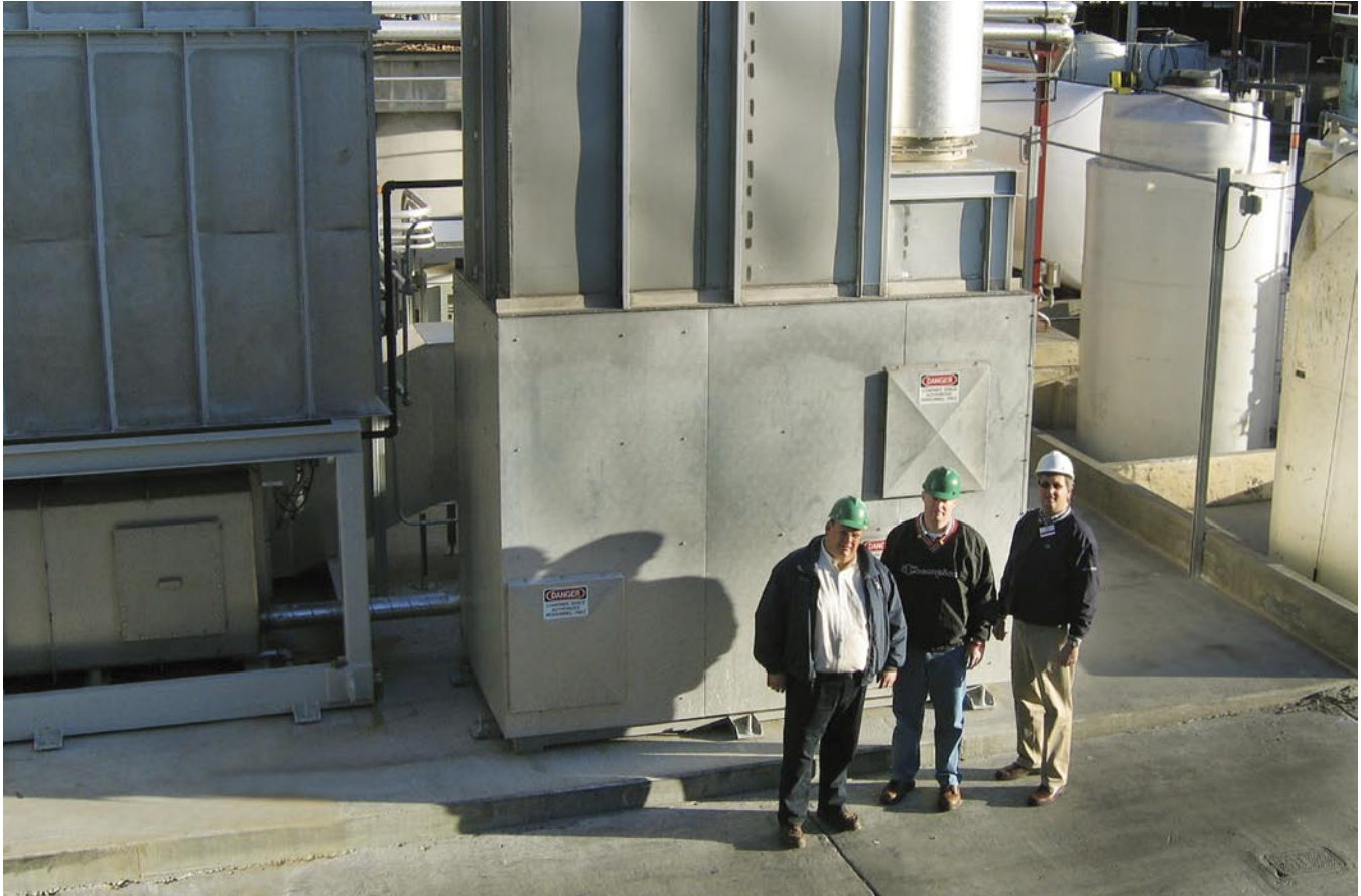
Mike Oliver (plant engineer), Mark Carlstrom (staff engineer) and Tom Holstrom (principal environmental engineer) in front of the RTO at Clougherty Packing Company's Vernon Avenue Plant.
